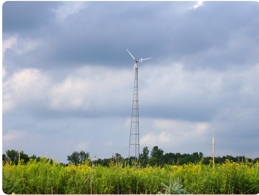
Small garden turbine (photo: CC BY 2.0, via Wikimedia Commons) — free, high site, guyed mast
